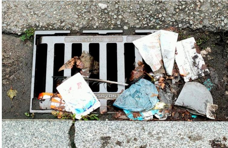
Figure 2. Sewer grate and plastic debris partially clogging a significant area of the inlet section (July 2021, German flooding).
